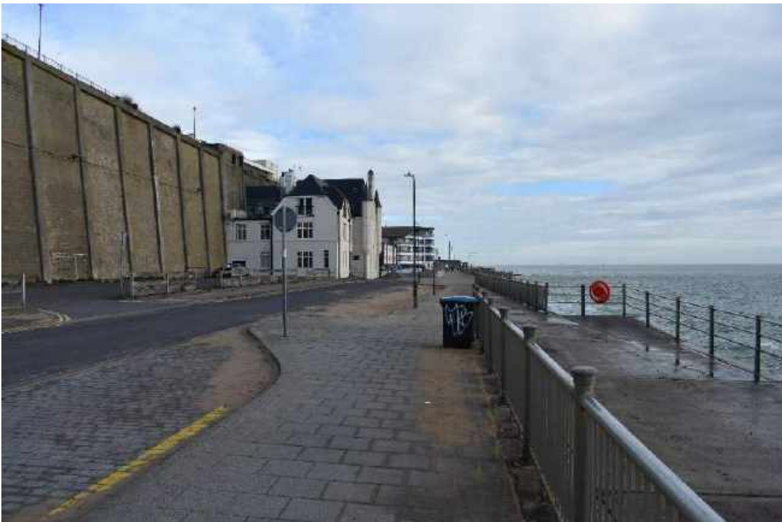
View north along Granville Marina
