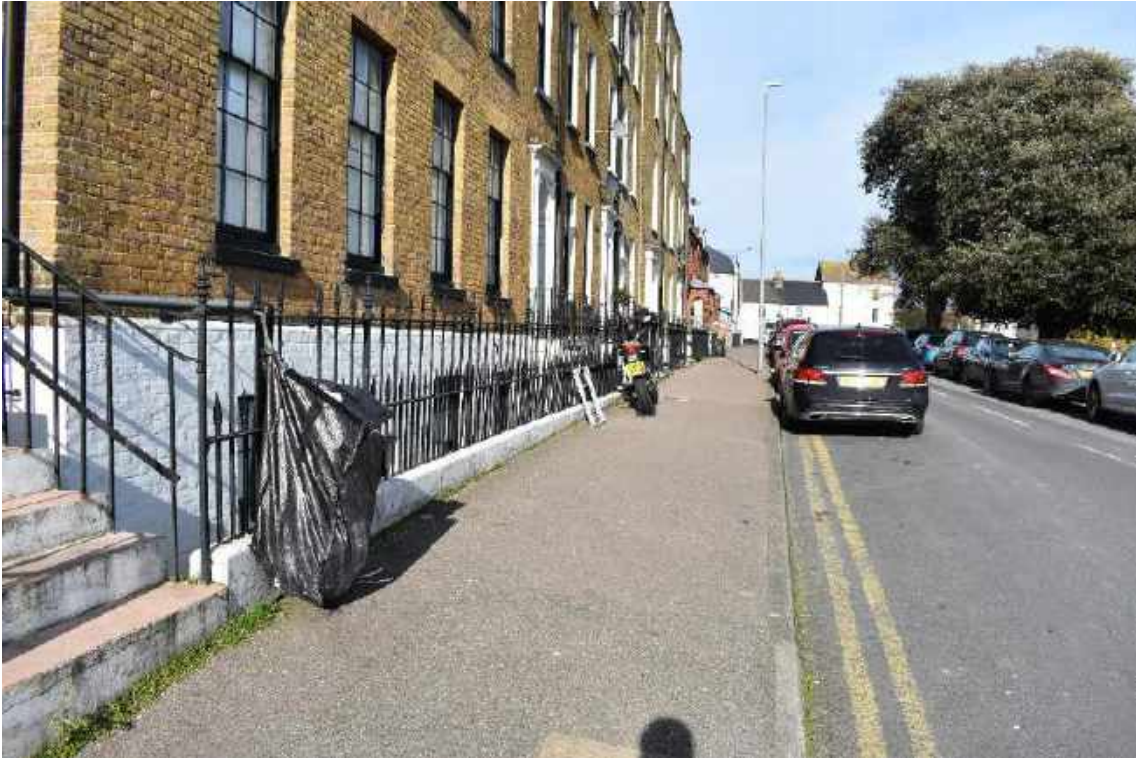
Iron railings on Chatham Place
