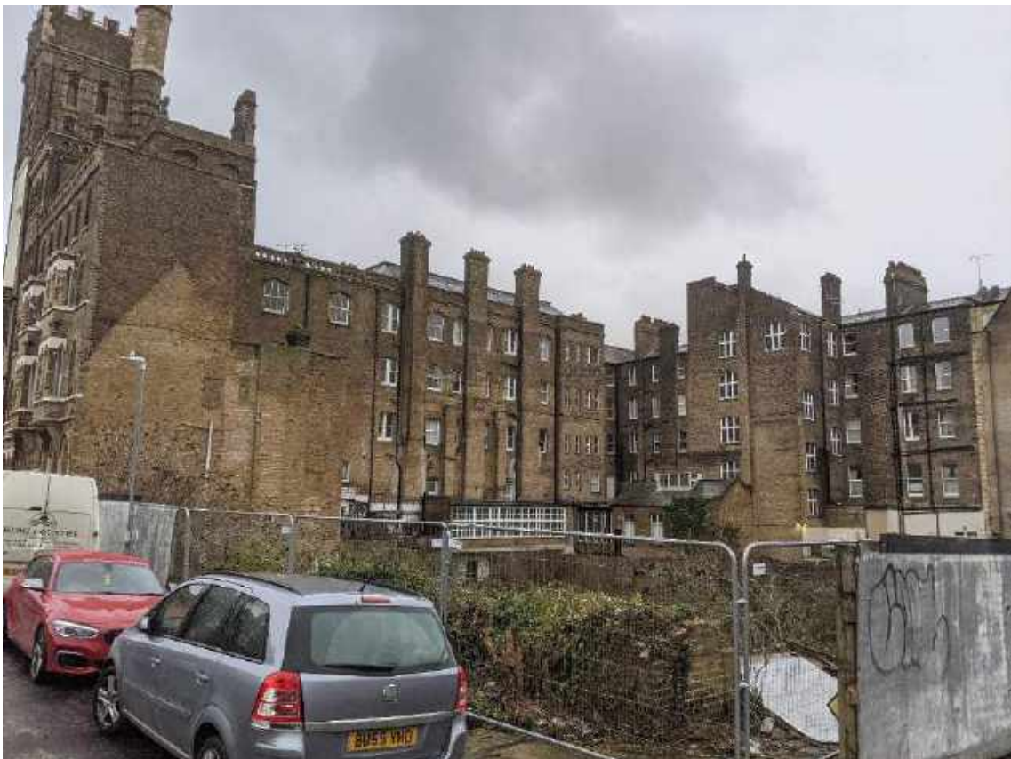
Vacant site behind the former Granville Hotel
