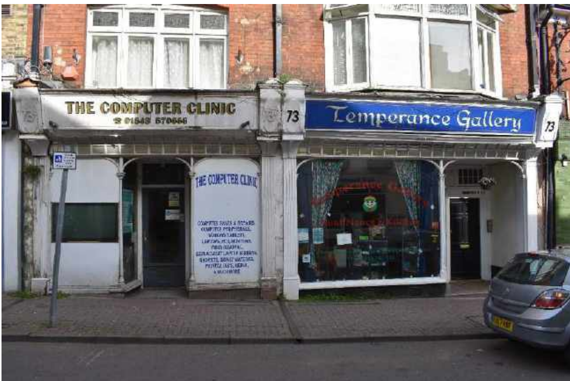
Historic shopfronts on the High Street
