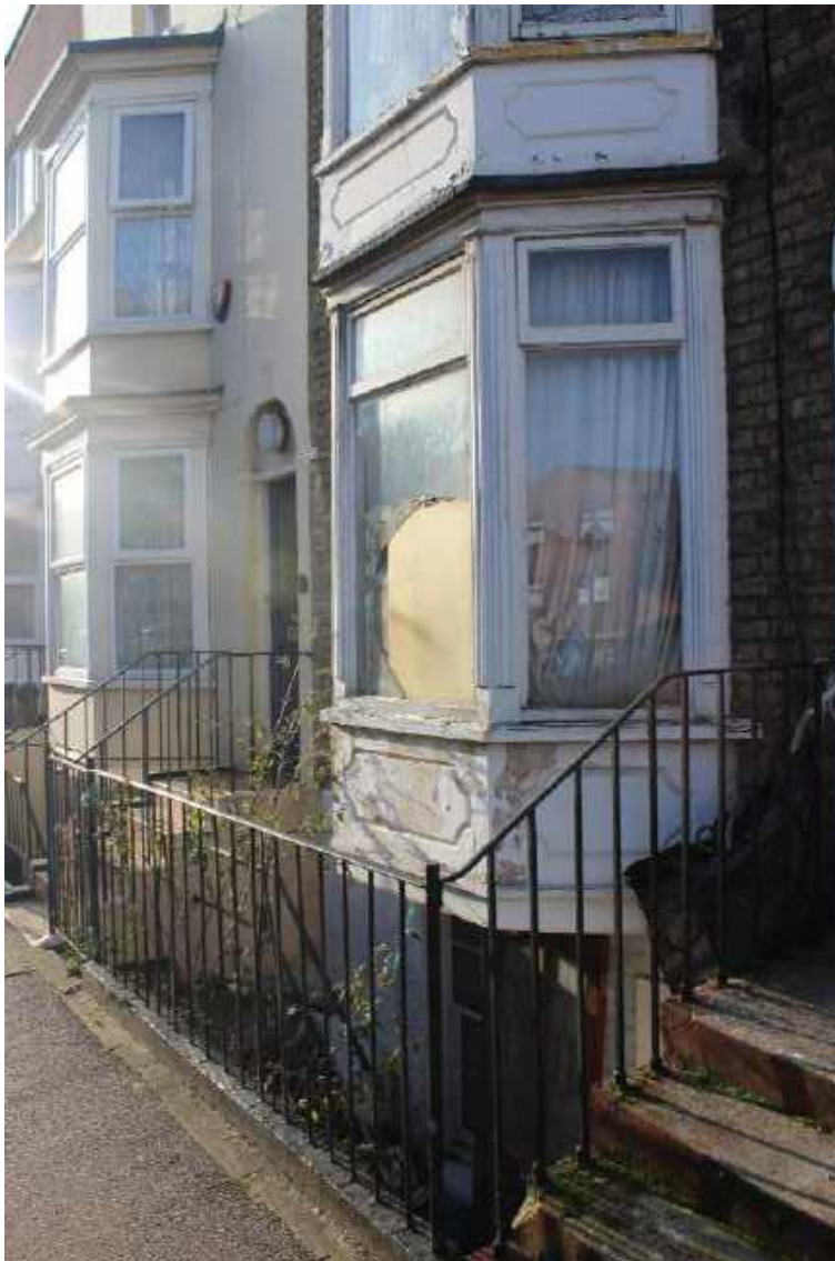
uPVC windows in historic townhouses
