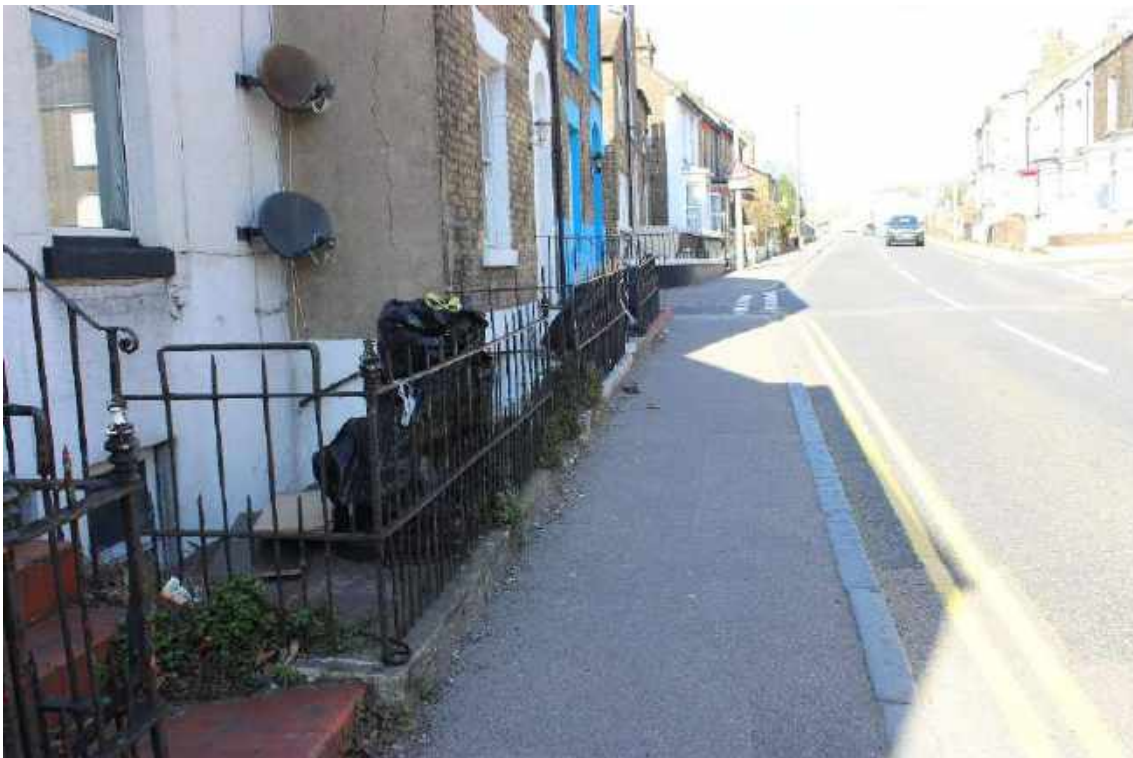
Iron railings in front of basement areas
