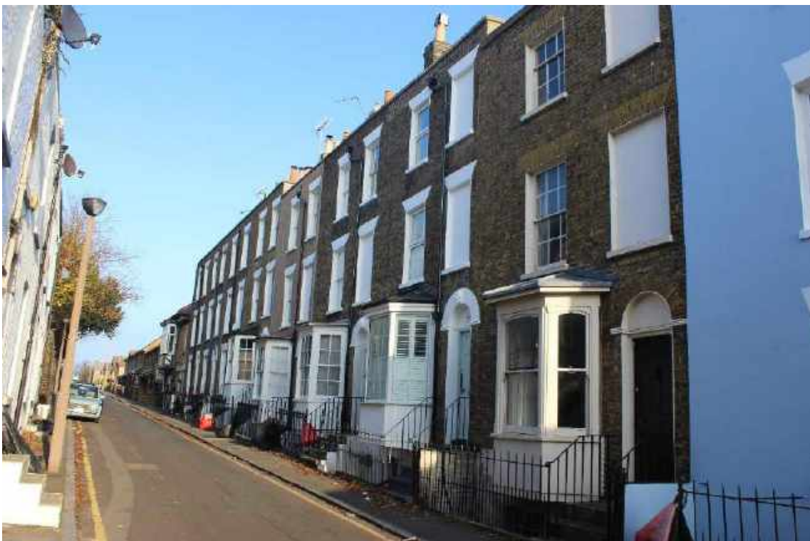
Canted bays and Classical proportions on Church Road
