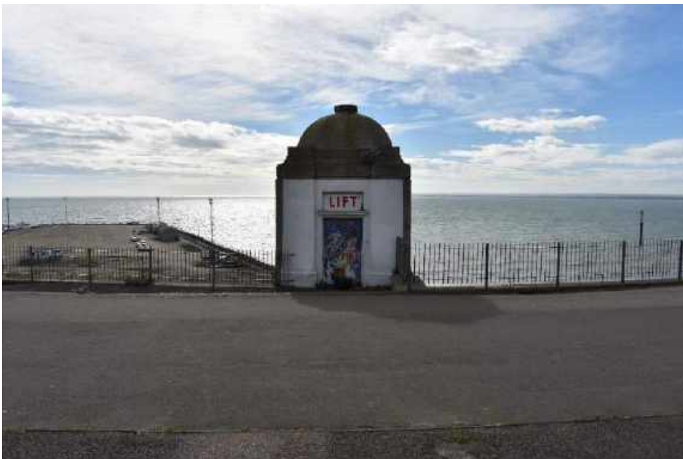
Lift at the western end of West Cliff promenade
