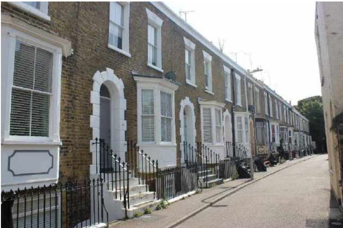
Two-storey, nineteenth-century terrace
