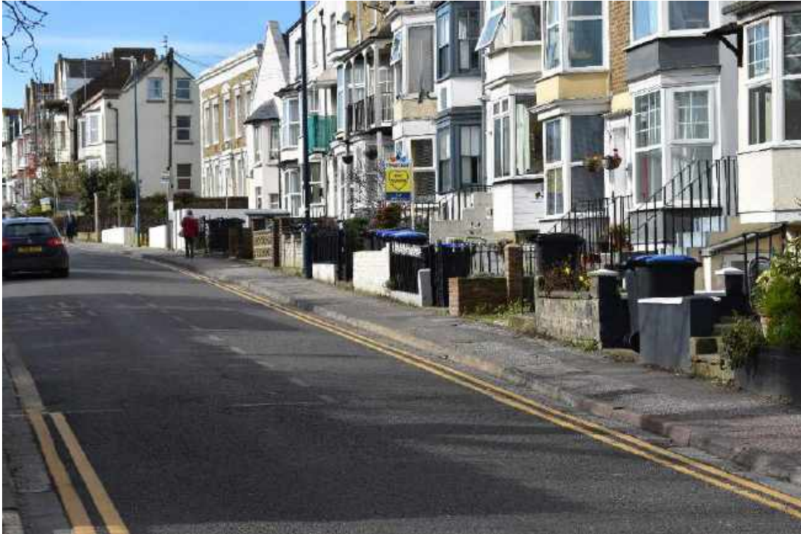
A wide variety of surviving historic features and later harmful additions
