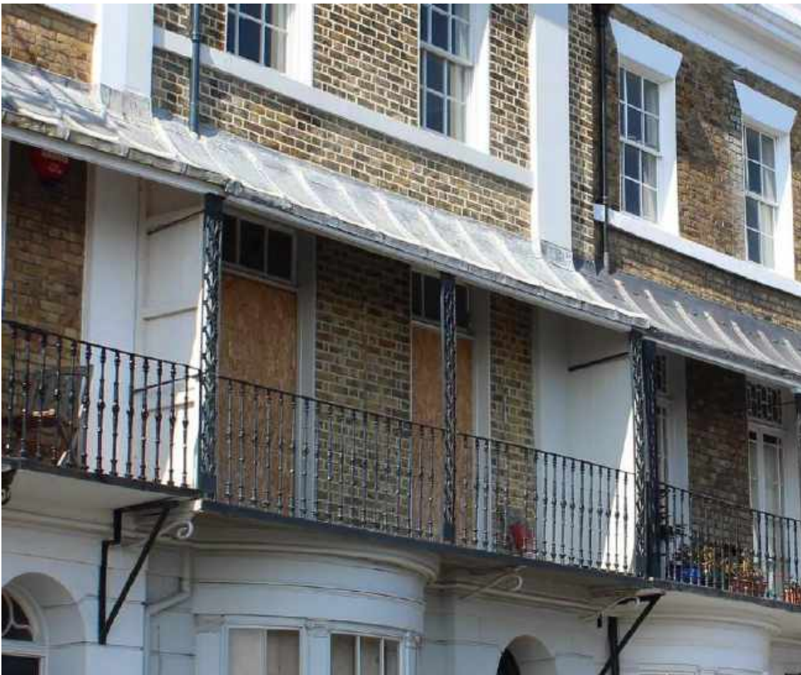
Iron verandah with lead roof, stucco details, brick in Flemish bond
