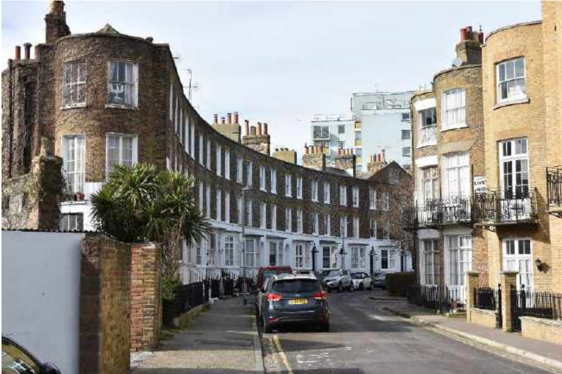
The crescent of Nos.1-19 Liverpool Lawn
