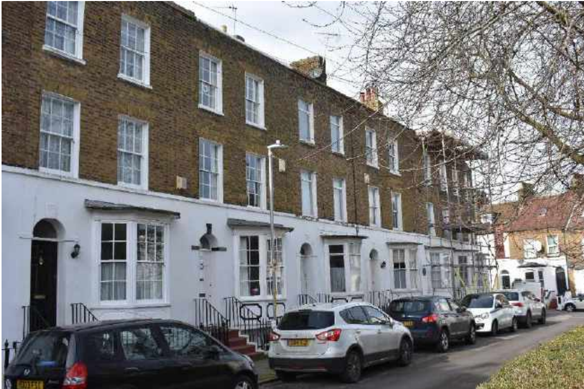
Stuccoed ground floors with canted bays, and many surviving historic timber sashes
