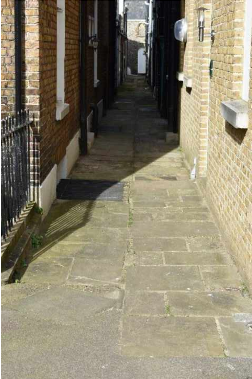
Retained stone flags along an alleyway in Character Area 6
