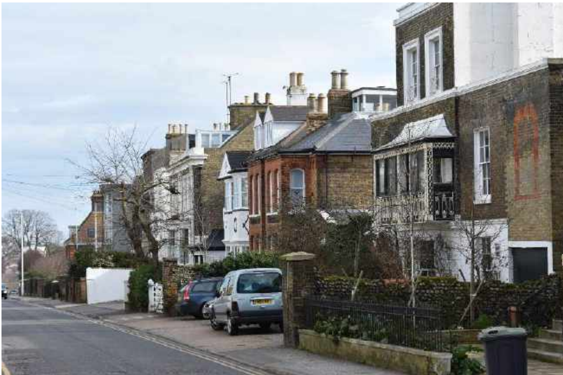
Detached villas at the western end of West Cliff Road
