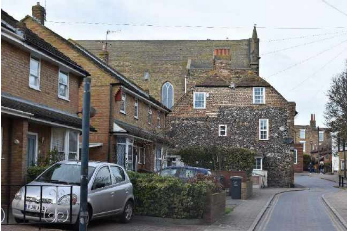
Flint used as a walling material in this eighteenth-century house on Meeting Street
