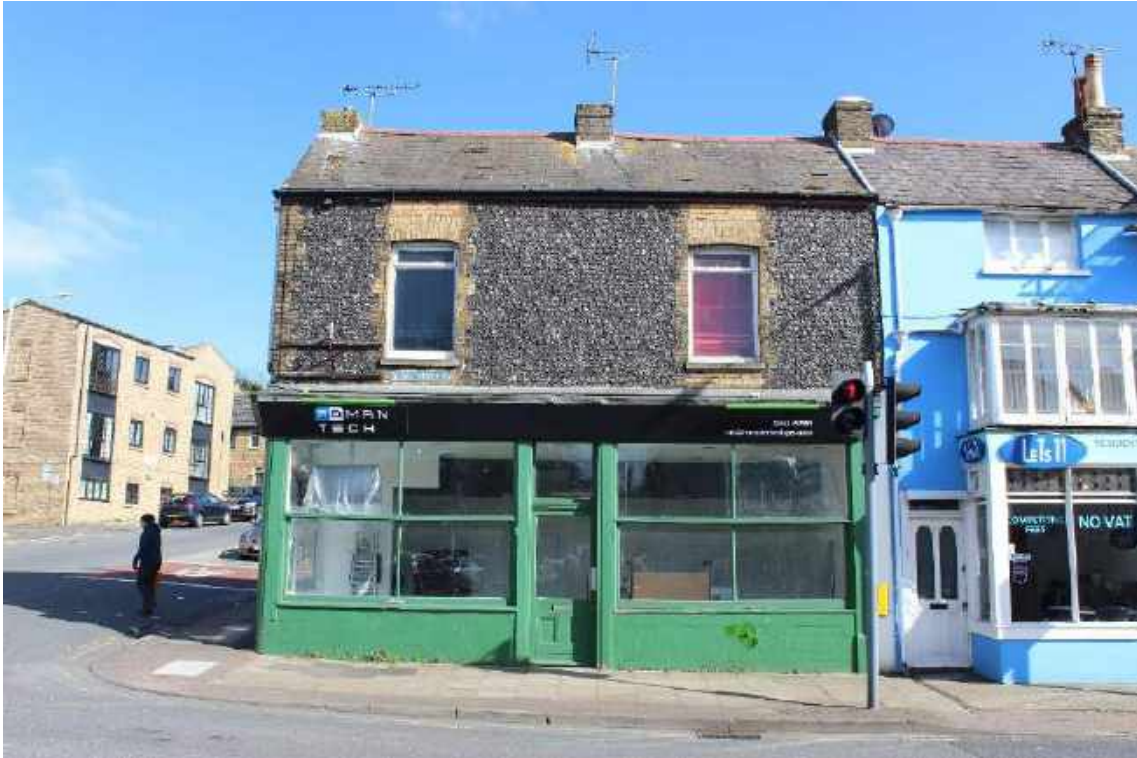
Knapped flint on the first floor and a timber and glazed shopfront on the ground floor
