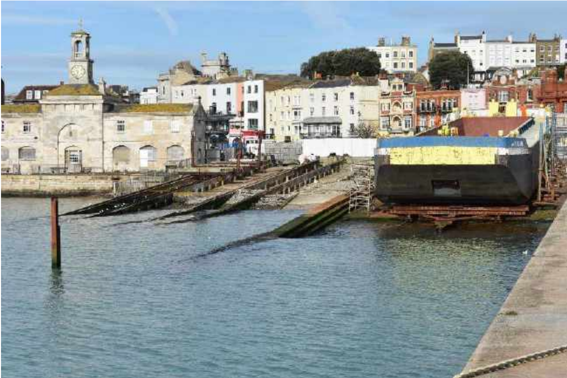
Nineteenth-century slipways viewed from the eastern harbour arm
