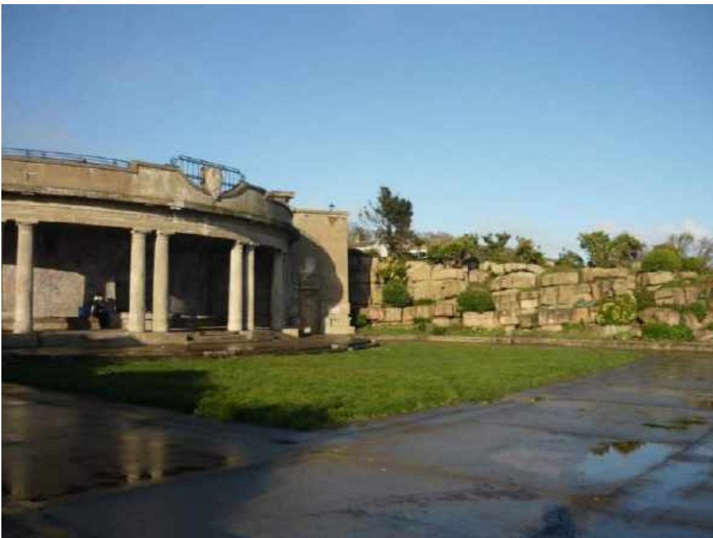
Strong landmark building with opportunity for better lighting
