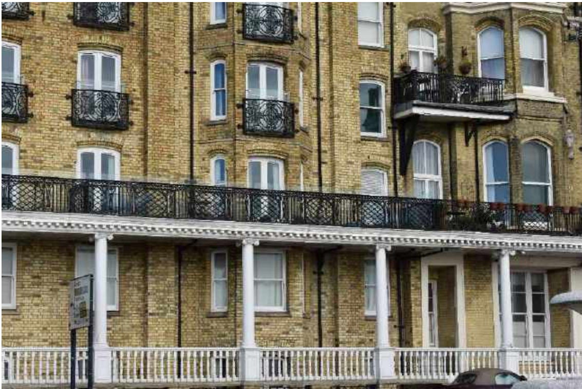
Brick detailing, iron balconies and canted bays onto the former Granville Hotel
