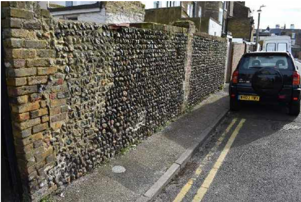
Flint and brick used as a boundary wall material on Hertford Street
