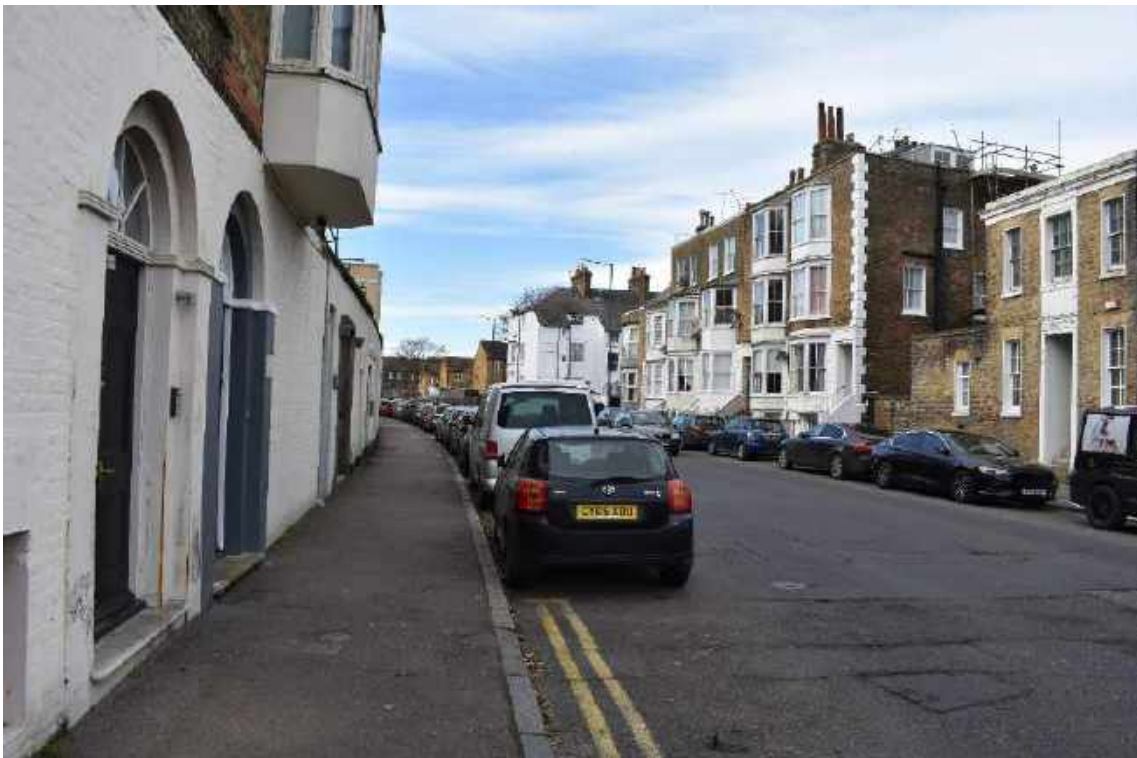
View west along St Augustine's Road
