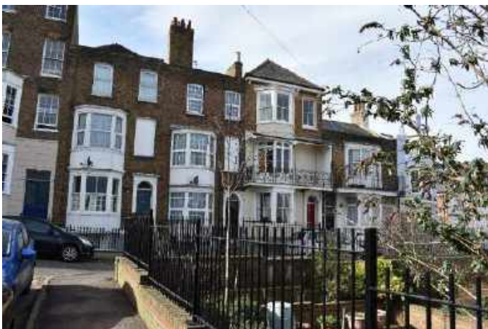
Varied use of a standard set of architectural forms and materials on Rose Hill
