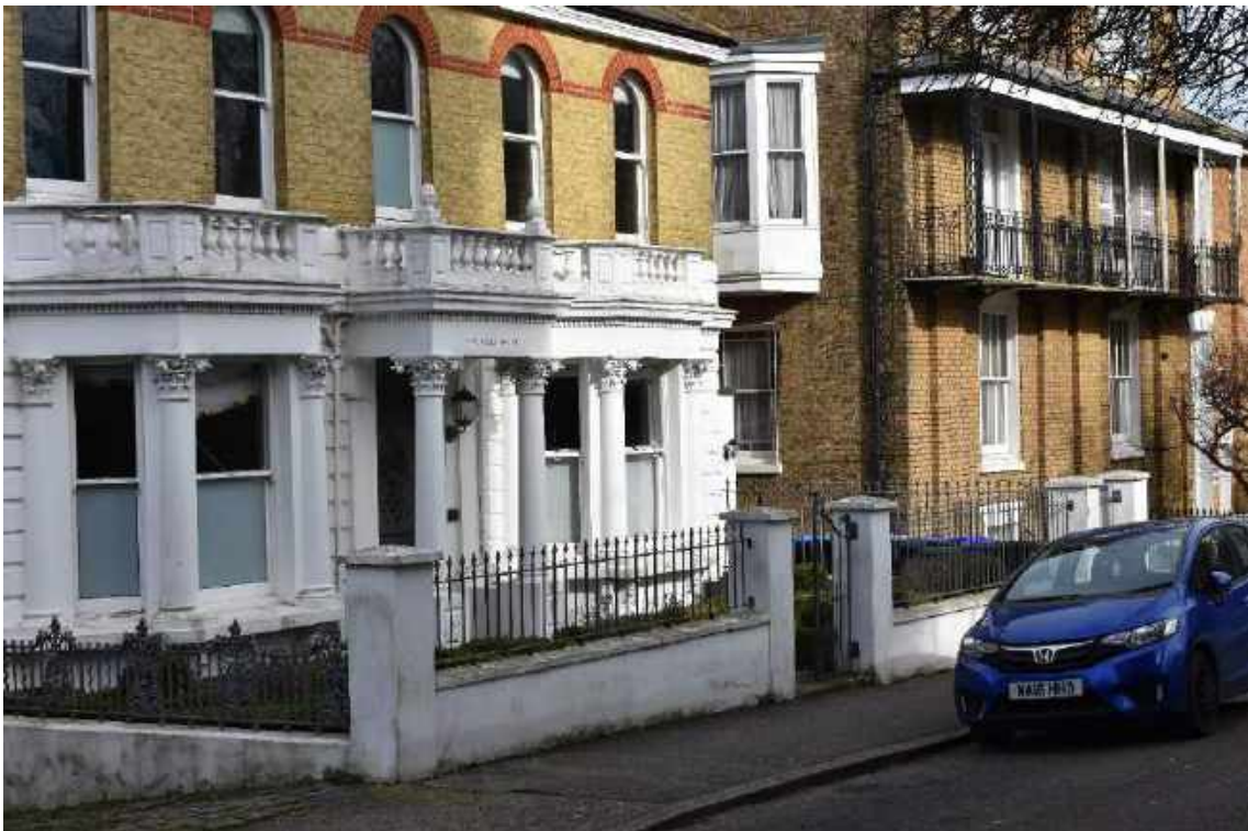
Rendered boundary walls with railings and terminating piers
