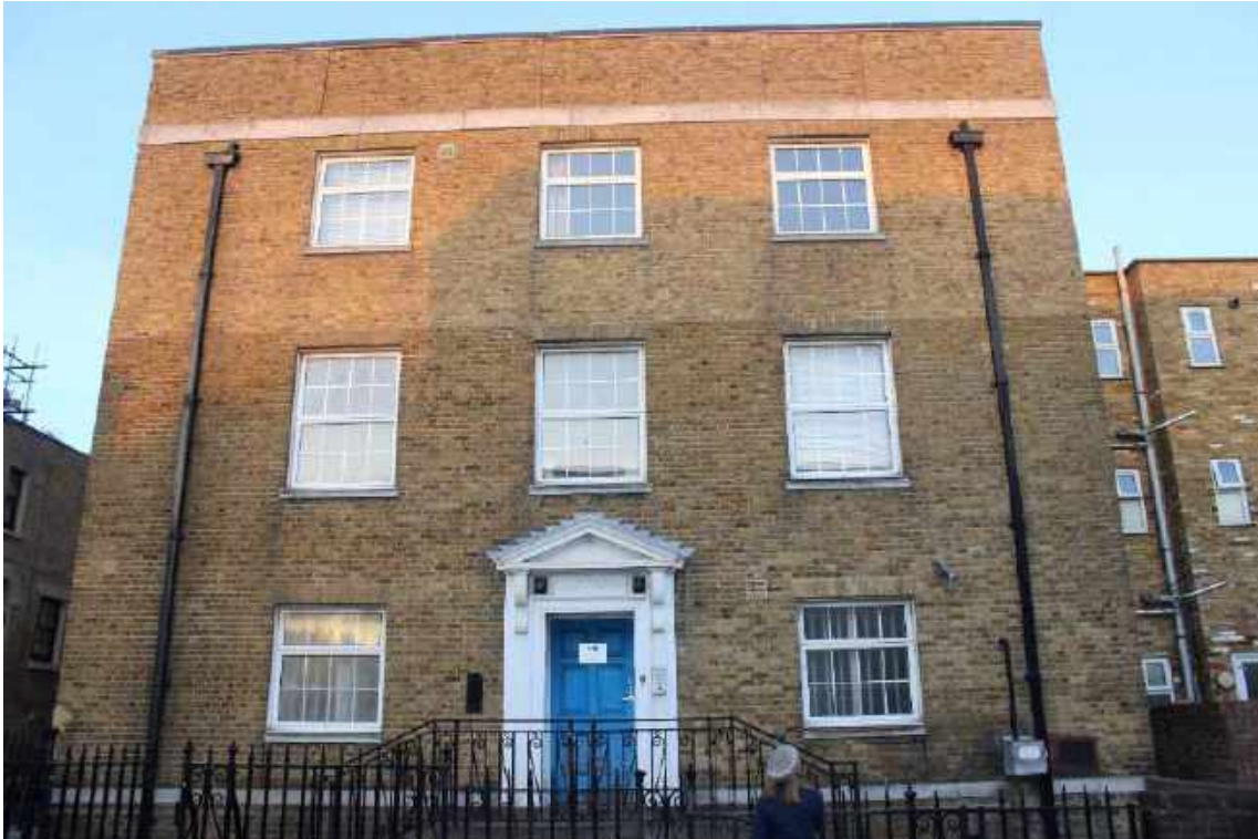
East elevation of the telephone exchange on Hardres Street
