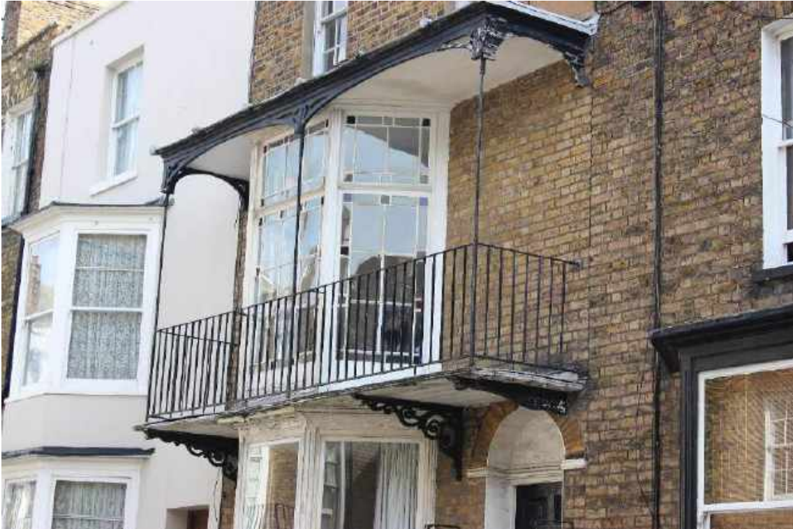
Iron veranda and bay windows
