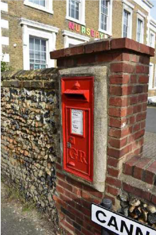
Historic wall-mounted letter box, West Cliff Road, set into a flint boundary wall
