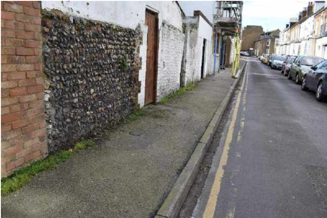
Flint used as a boundary wall material on Albert Street
