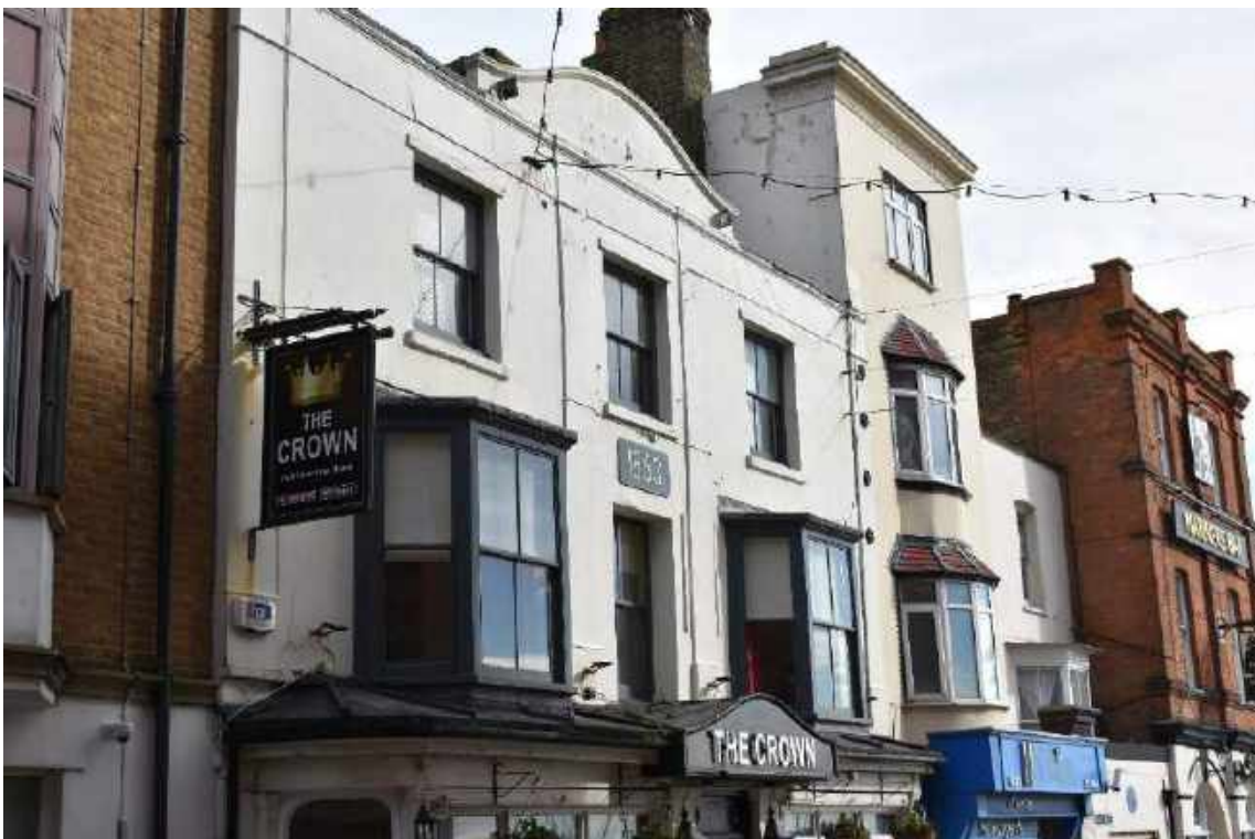
First floor bay windows on York Street
