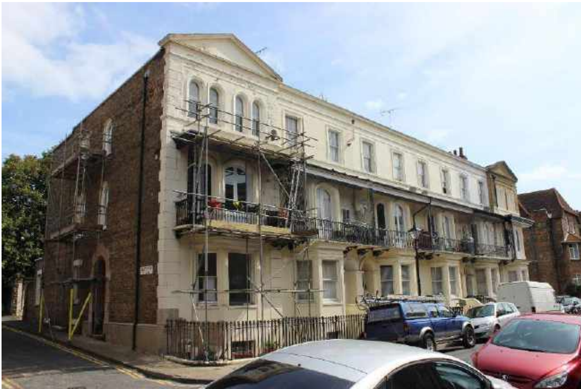
Listed terrace on Augusta Road
