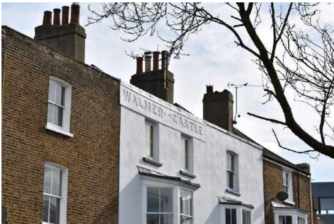
Historic building names inscribed into stucco or stone can enrich the streetscape
