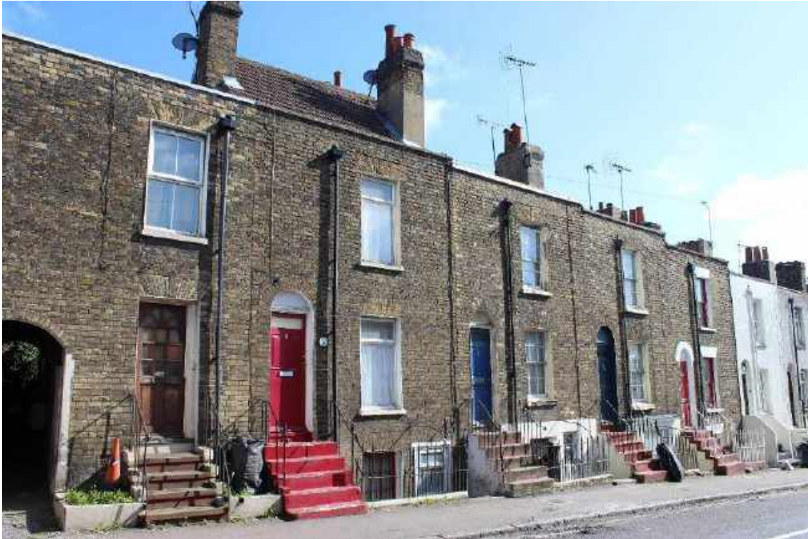
Late-eighteenth or early-nineteenth century terrace on King Street
