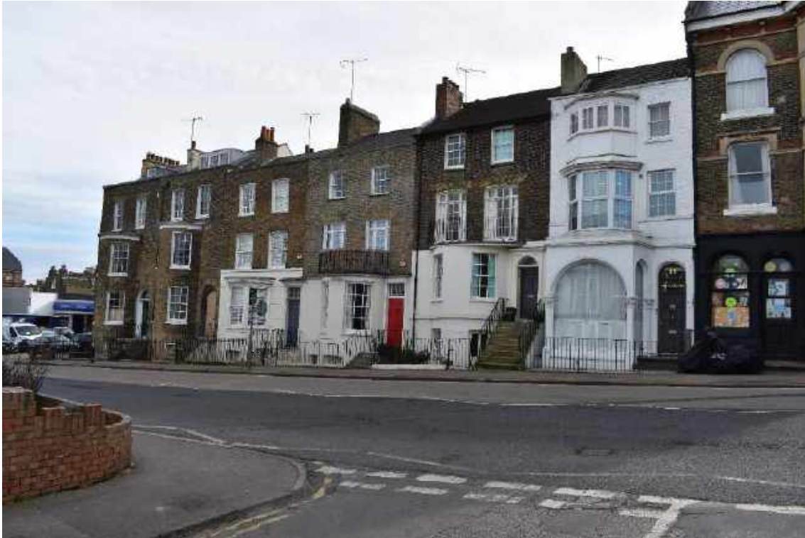
Early-nineteenth-century terrace at the eastern end of West Cliff Road
