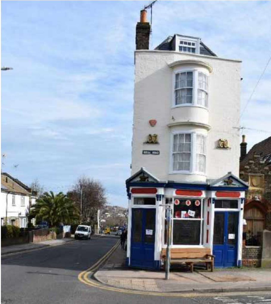
The prominent western elevation of the Artillery Arms
