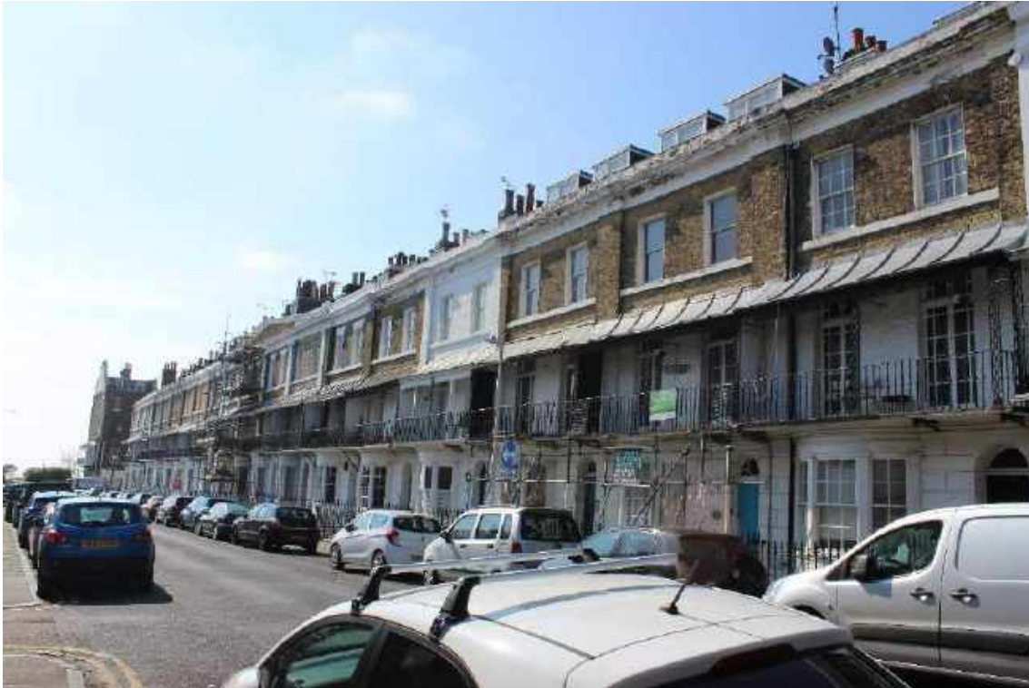
Three-storey terrace with Classical detailing
