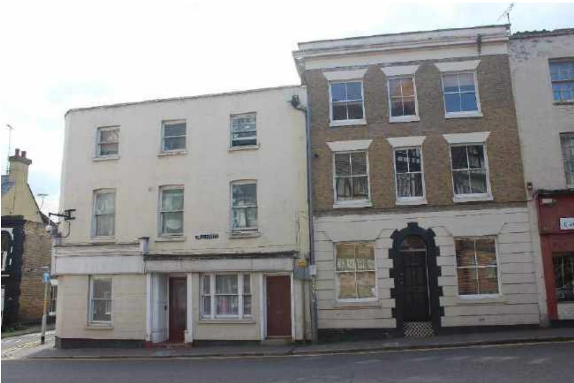
Houses built hard up to the pavement on High Street
