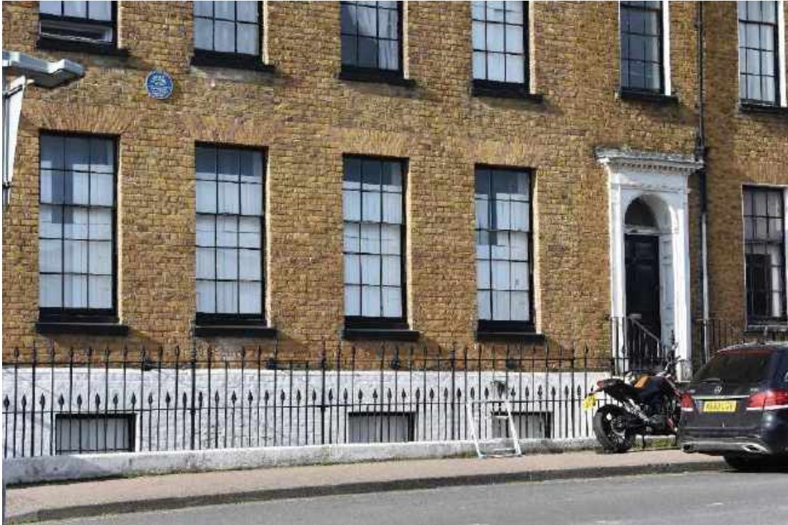
Historic timber sashes and door surrounds on Chatham Place
