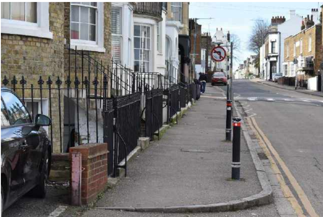
Iron railings around front basement areas on West Cliff Road
