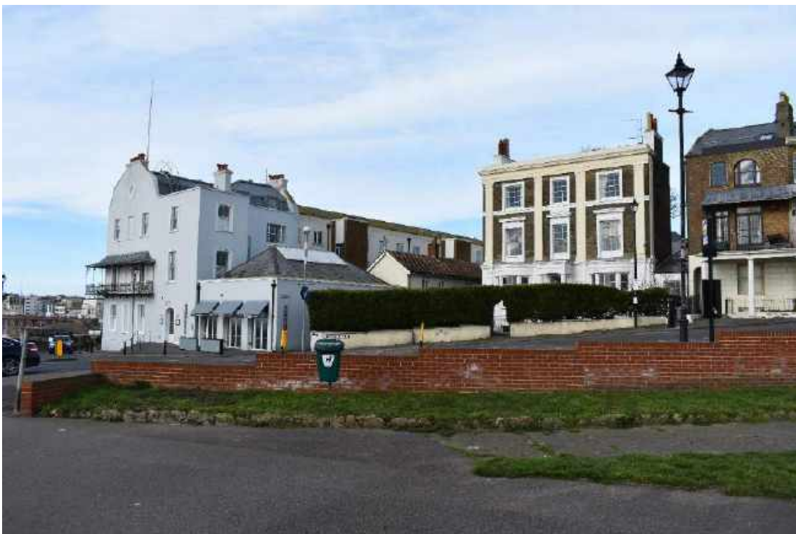
Stucco render used as a primary facing material and for embellishment
