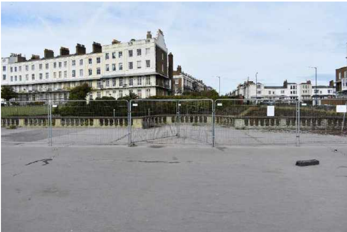
The fenced-off sunken gardens of West Cliff Hall
