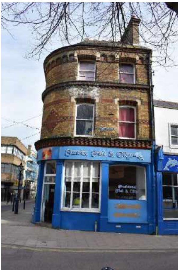
This nineteenth-century building on Queen Street is a focal point of views due to its prominent corner location and fine architectural detailing.
