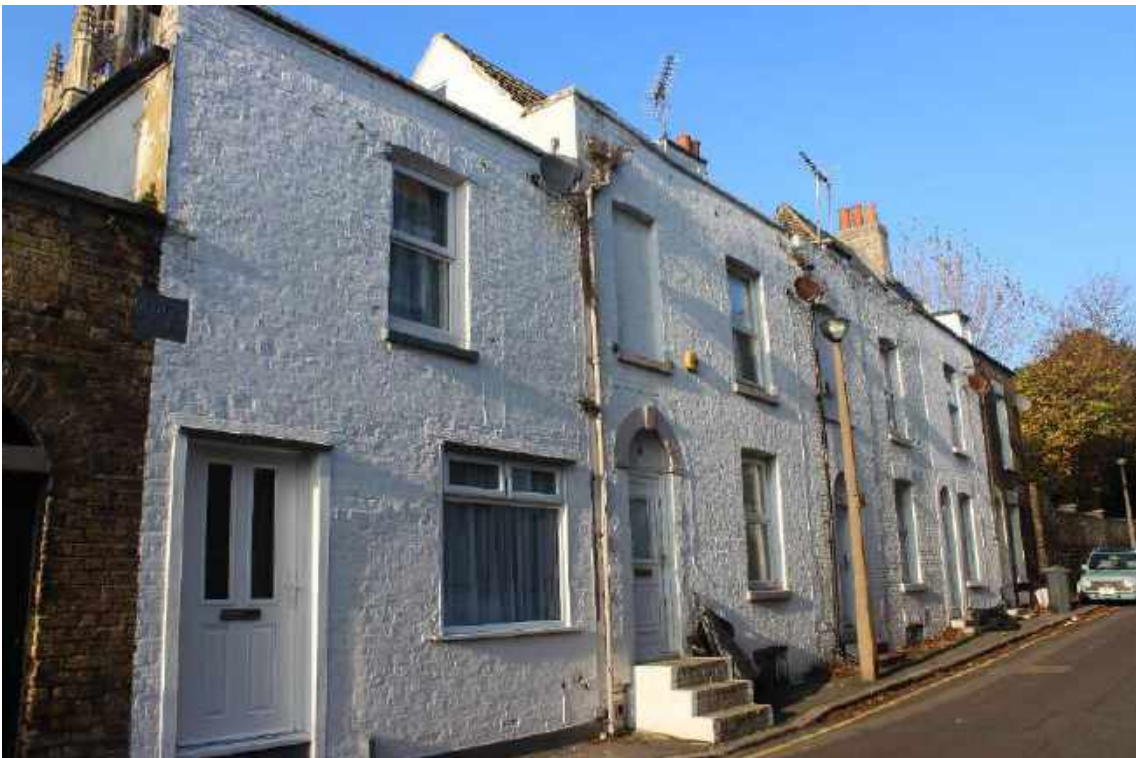
Buildings hard up to the pavement on Church Road
