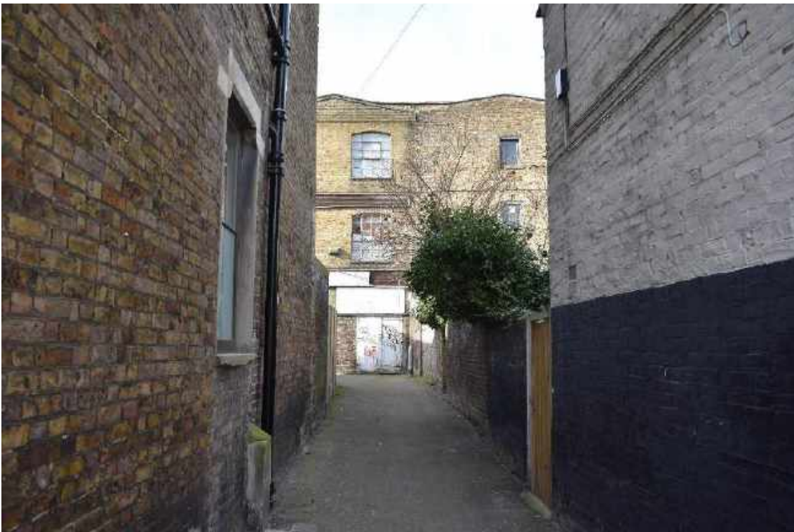
Dilapidated light industrial building on Chapel Place Lane
