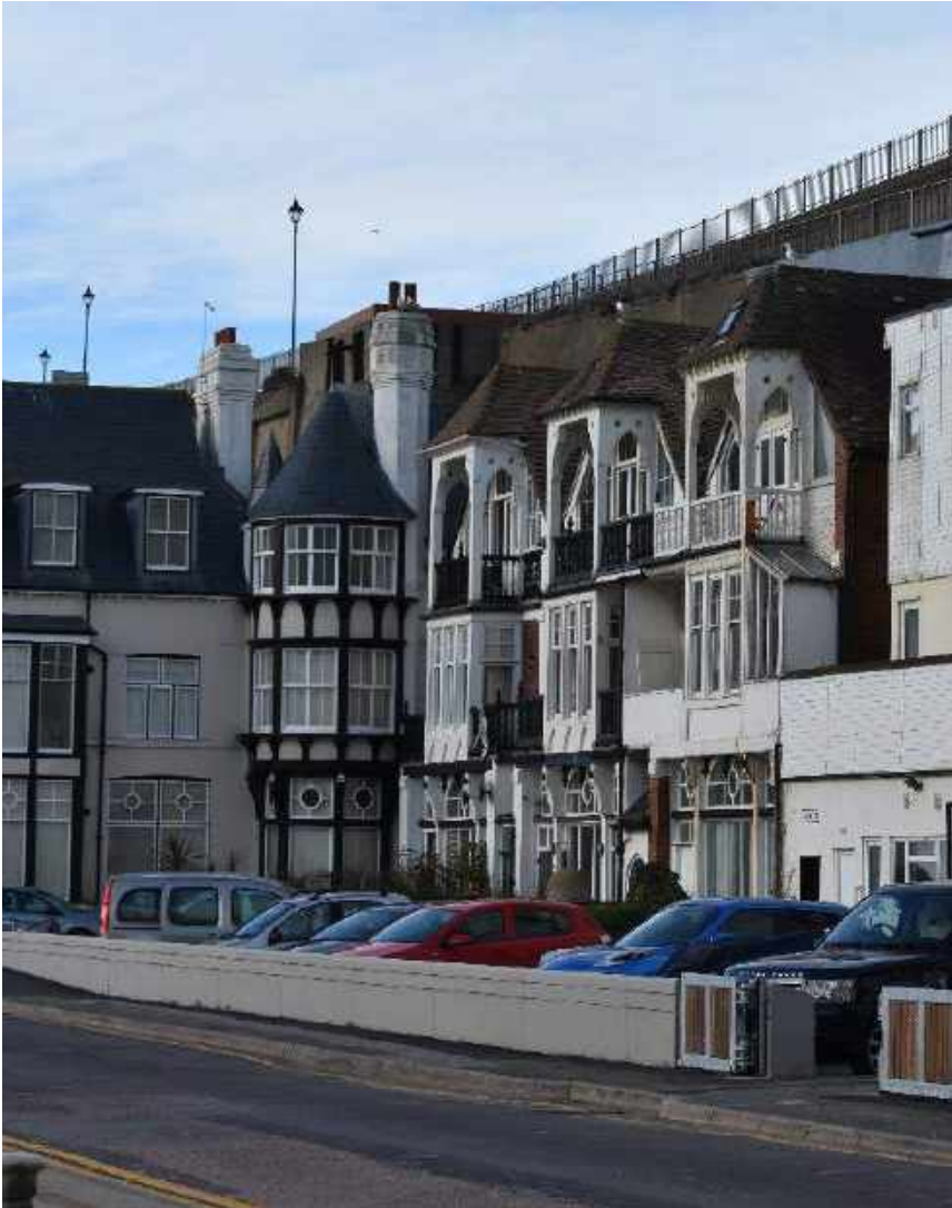
Listed nineteenth-century shops and houses at Granville Marina
