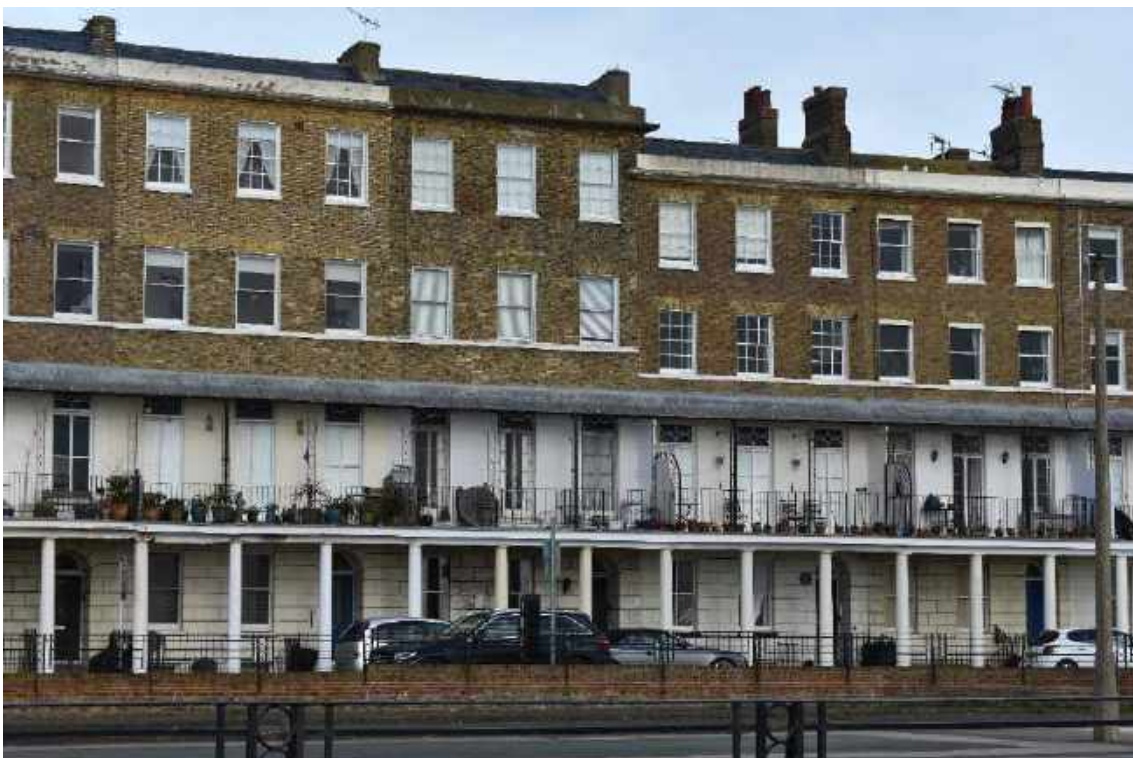
Brick, first-floor verandahs and ground-floor colonnade at Wellington Crescent
