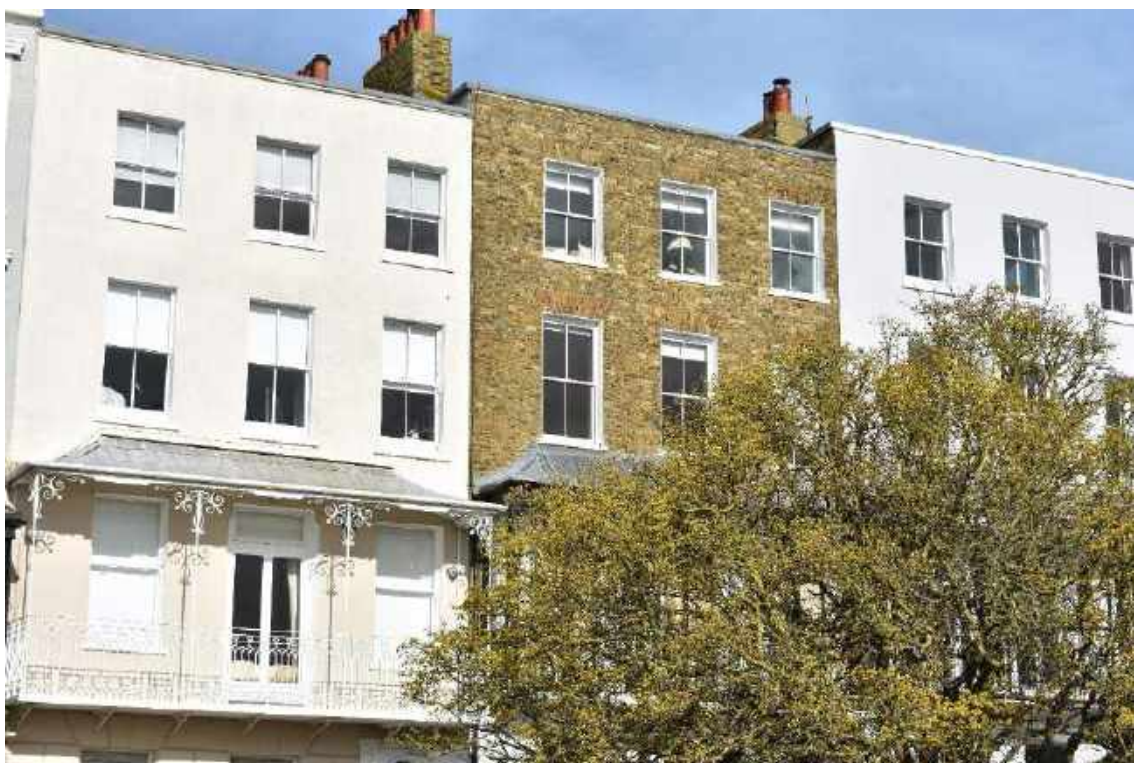
Townhouses on Albion Place with historic timber sashes and iron verandas
