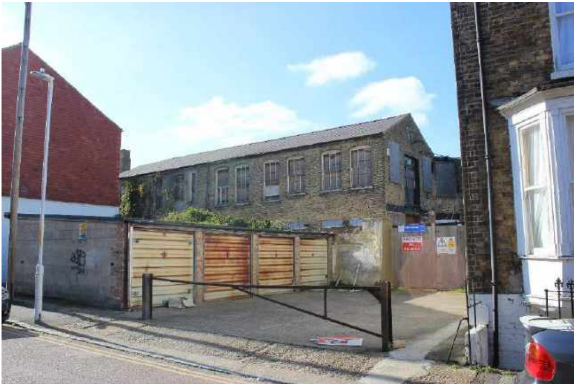
Former industrial workshops north of Townley Street
