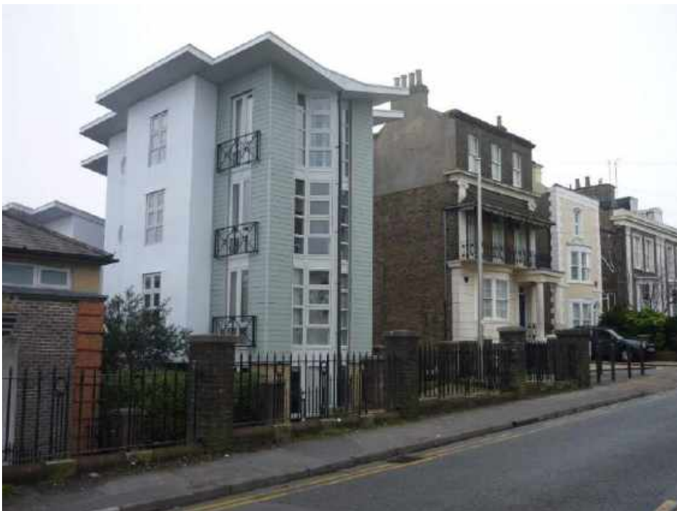
Unresponsive to locally distinctive historic context
