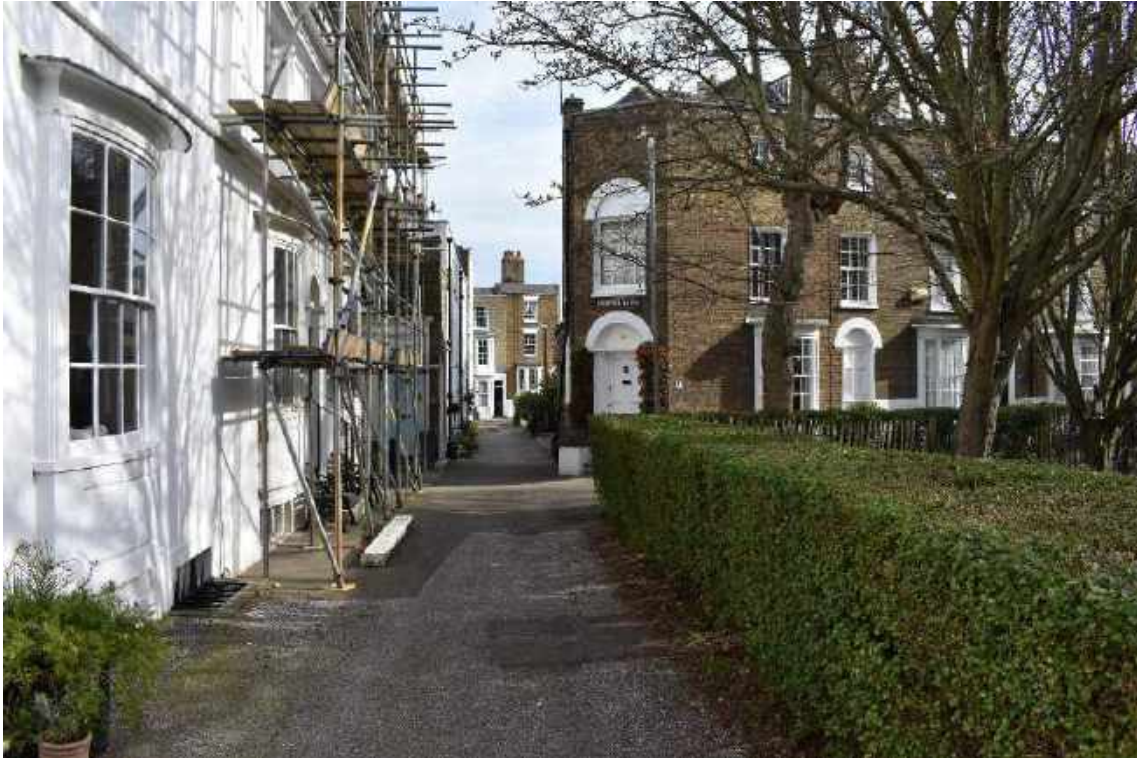
View east along the very narrow north side of Liverpool Lawn
