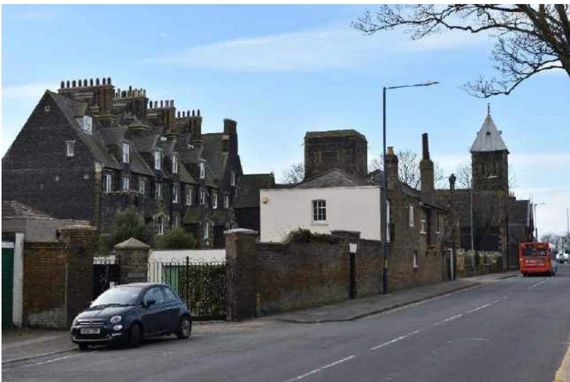
Extensive use of knapped flint on Chartham Terrace and St Augustine's Church
