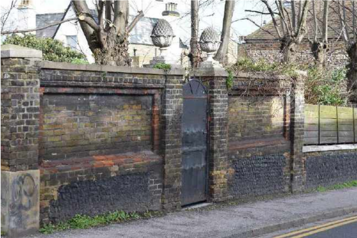
Tall brick boundary walls on West Cliff Road
