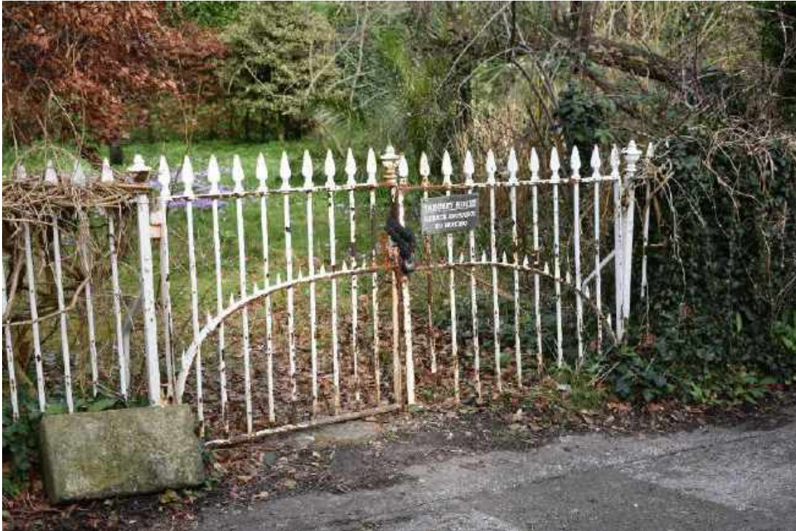
Iron railings on Vale Square Gardens
