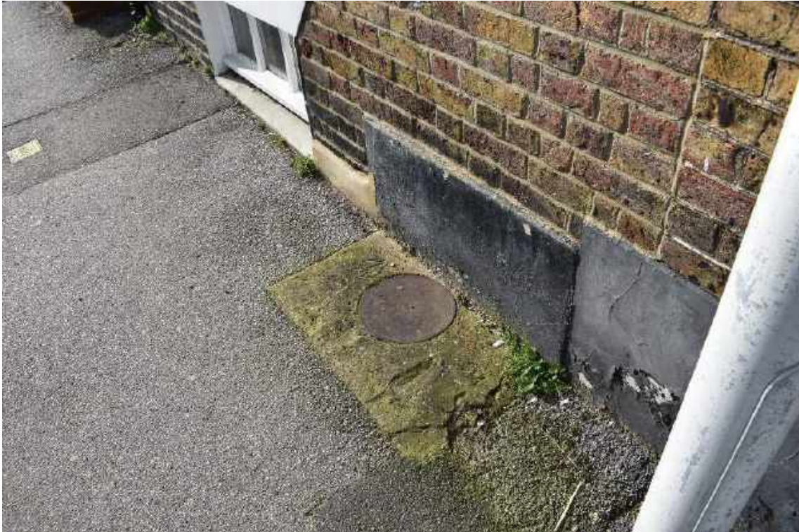
Coal chute cover within a retained stone slab on Chapel Place
