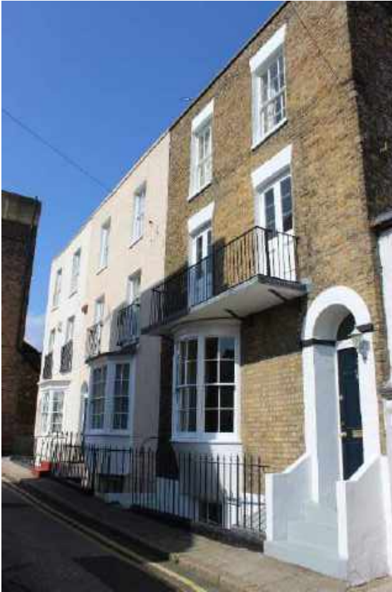
Iron railings around front basement areas
