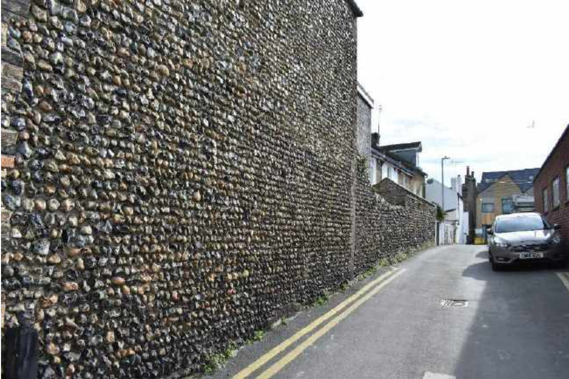
Coursed, unknapped flint used as a walling material on West Cliff Road
