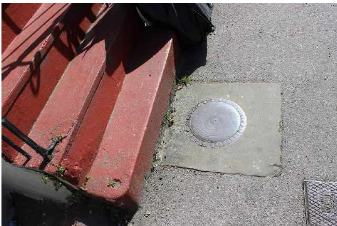
Coal chute cover on King street
