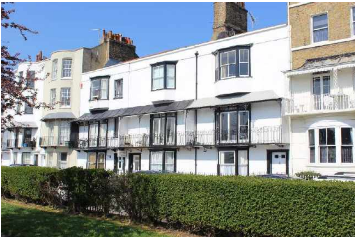
Fully rendered terrace with timber canted bays to all floors and iron verandahs
