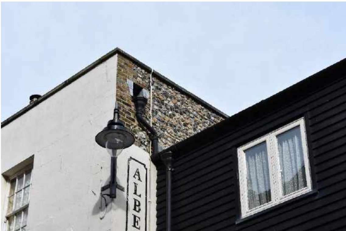
Flint used in the flank wall of a building on York Street
