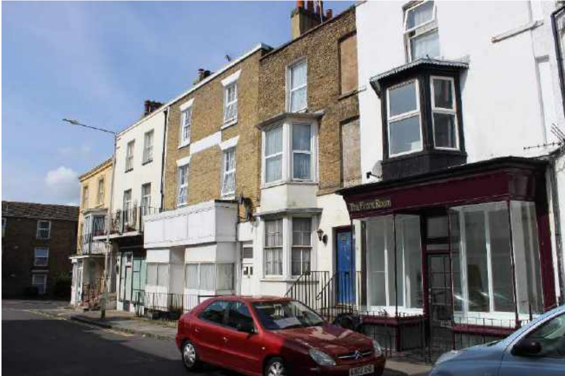
Retained historic shopfronts
