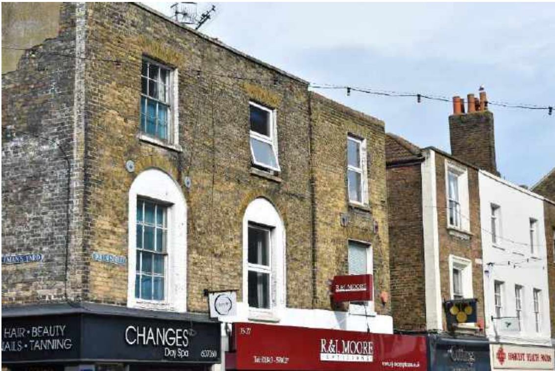
Buff brickwork and simple Classical detailing on early-nineteenth-century buildings on Queen Street
