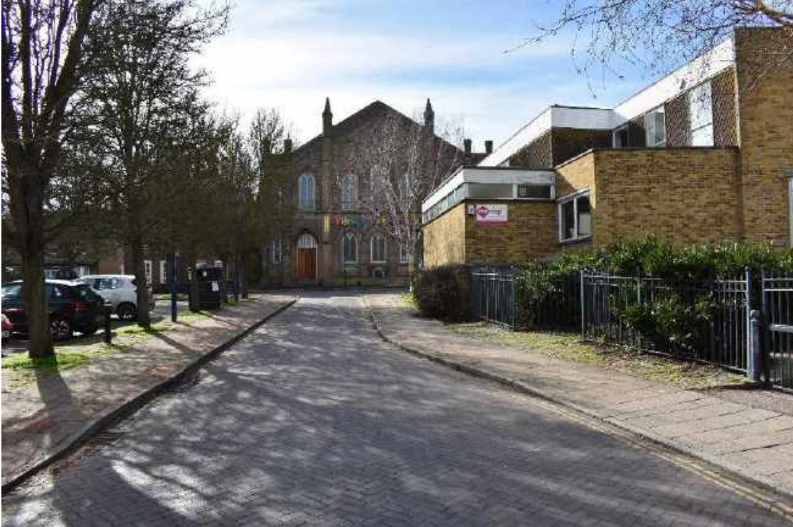
View of the former Congregational chapel at the west end of Meeting Street
