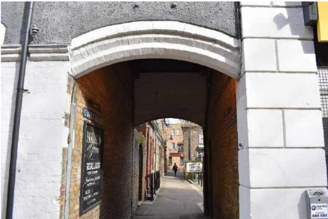
Passage through to Charlotte Court from York Street
