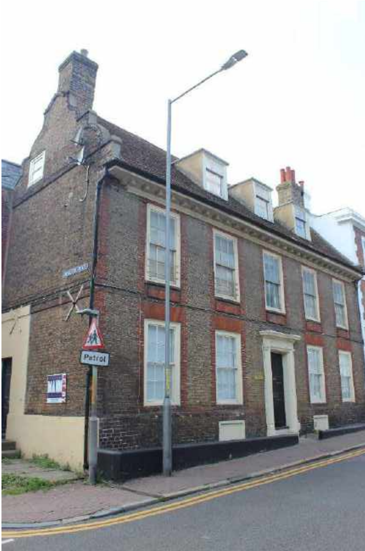
The eighteenth-century Monkton House has lost its iron railings but retains the masonry base
