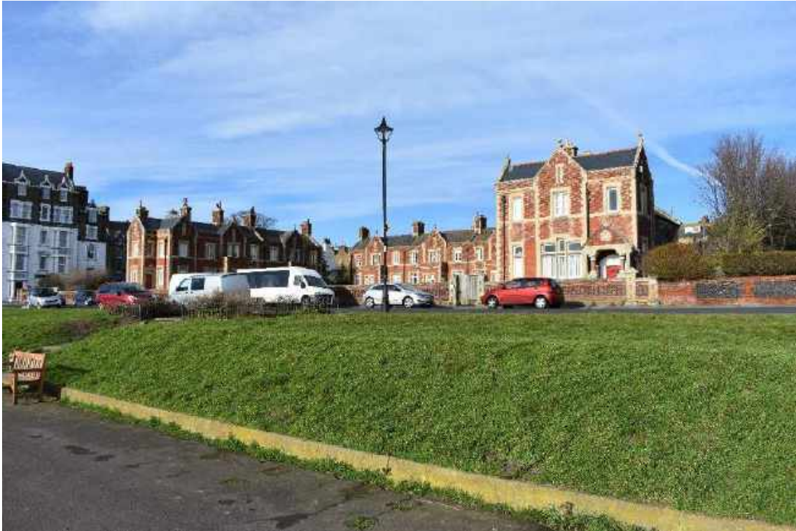
Former Coastguard station
