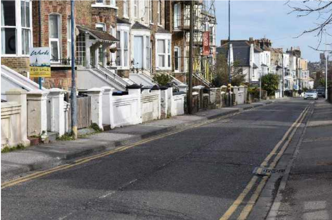
Rendered boundary walls with terminating piers
