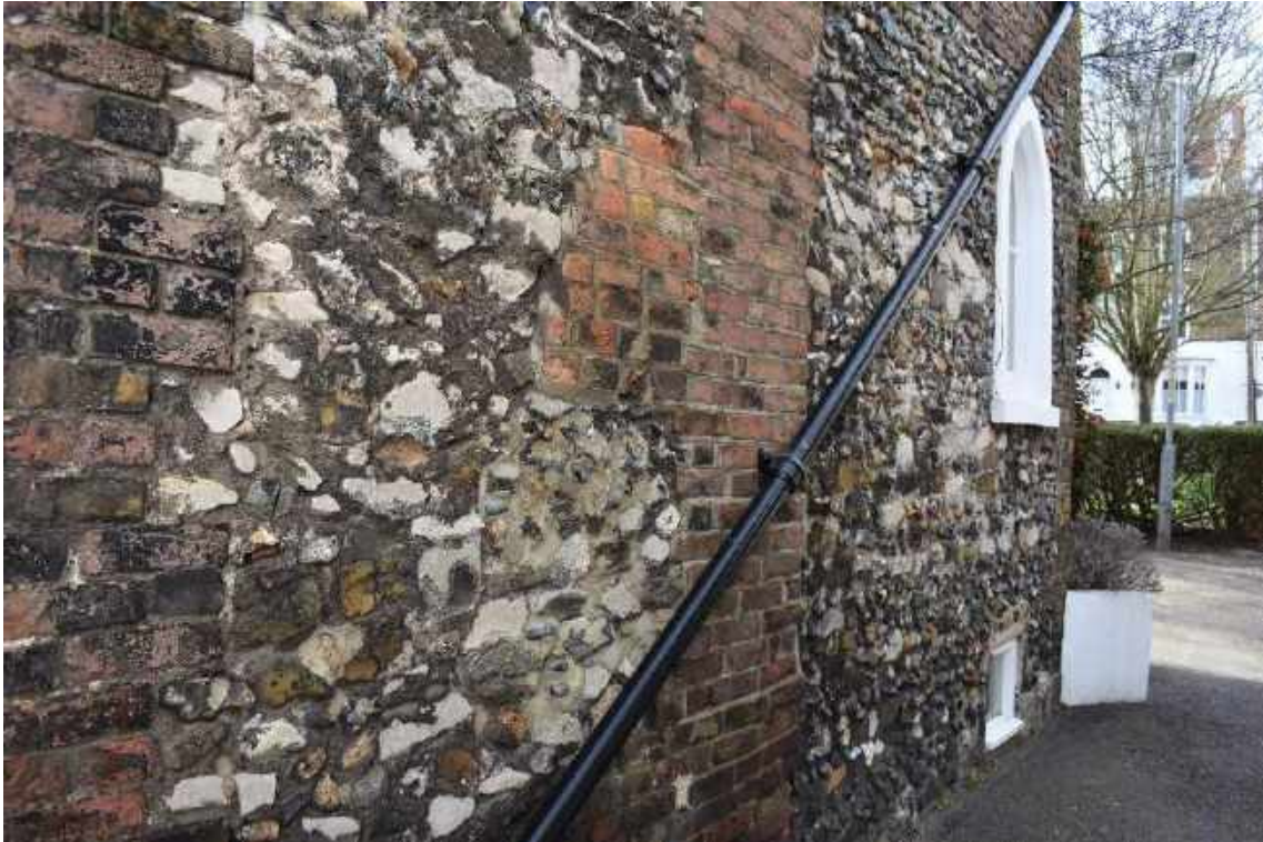
Flint, rubble and brick used as walling materials on Liverpool Lawn
