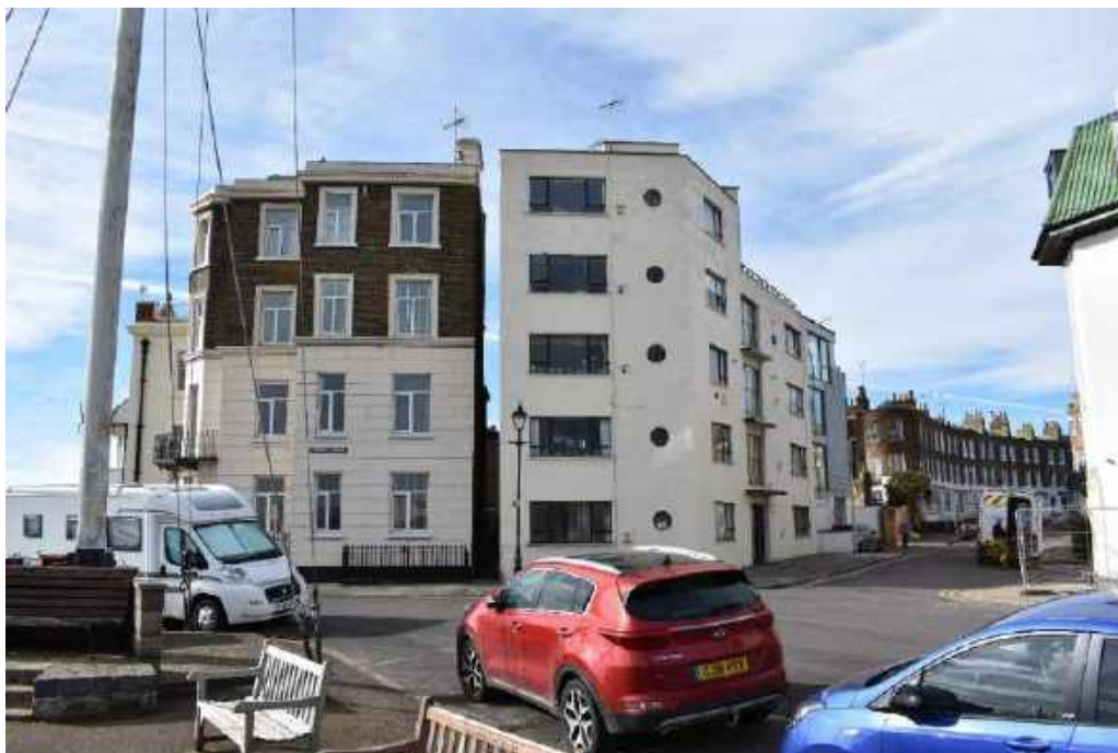
Prospect Court, a twentieth-century addition which detracts from the character and appearance of the conservation area
