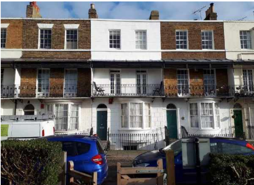
The verandah provides shading to the tall windows on the first floor of these fine town houses. The timber louvres that extend this shading are a common feature to the local vernacular.
