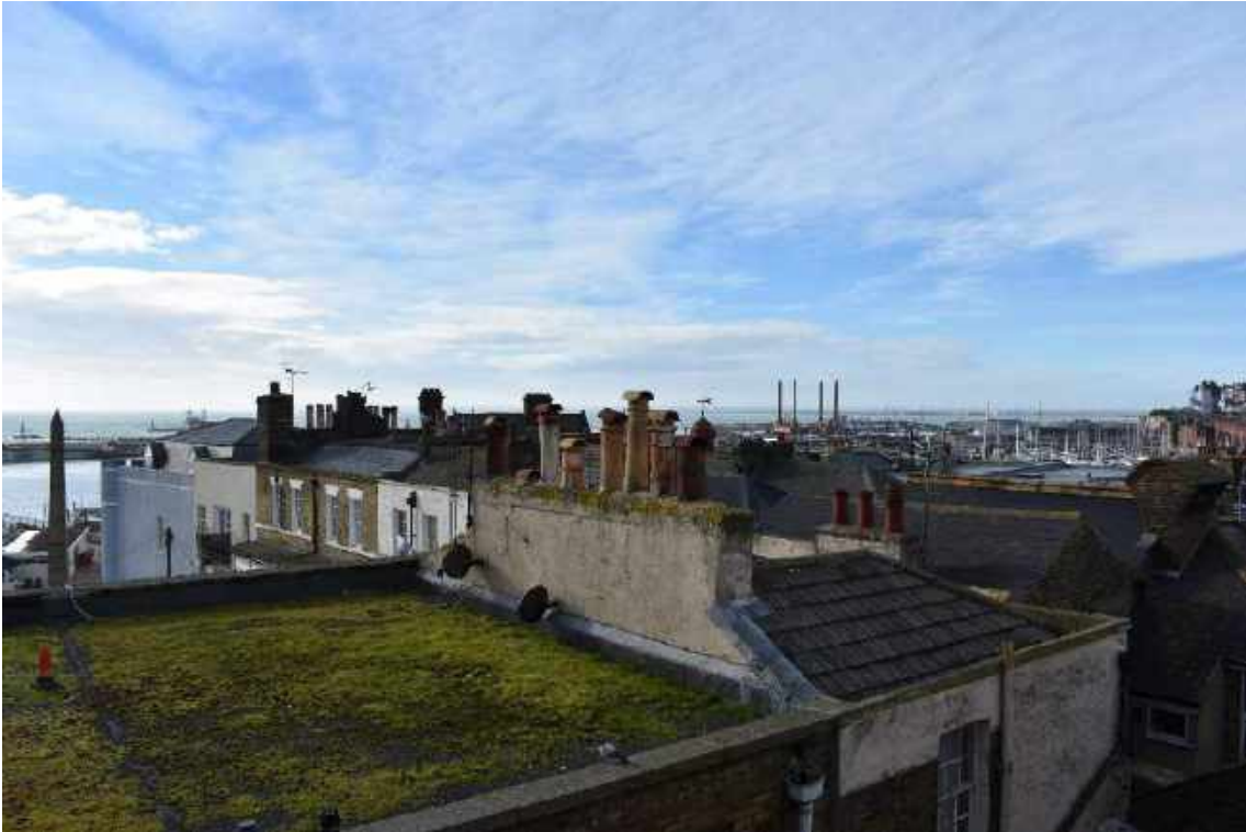
The evocative roofscape views gained from the top of Madeira Walk
