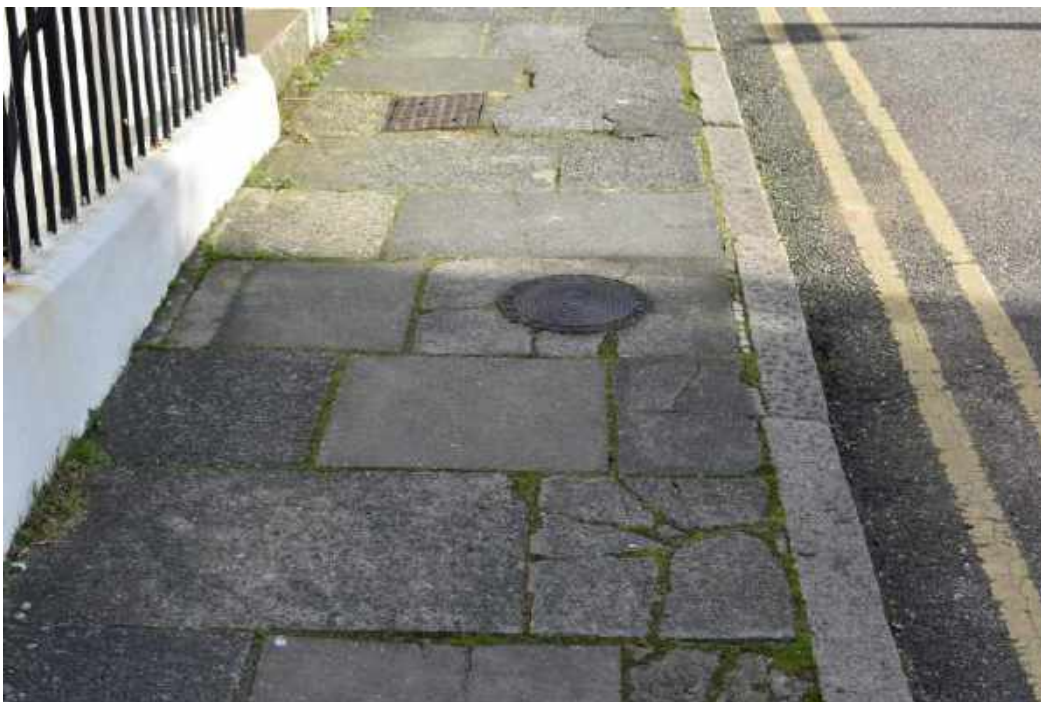
Coal chute cover on Albion Place
