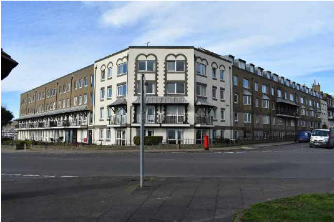
Homefleet House, at the junction of Victoria Parade and Augusta Road
