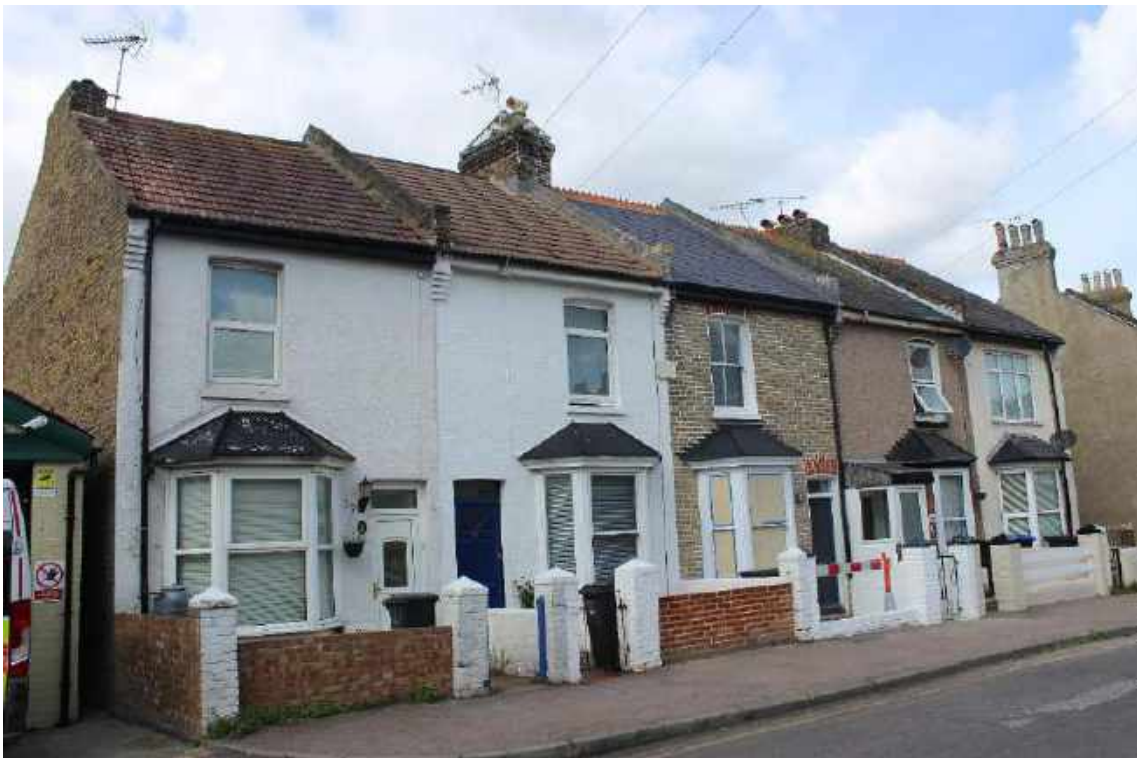
Loss of original features
