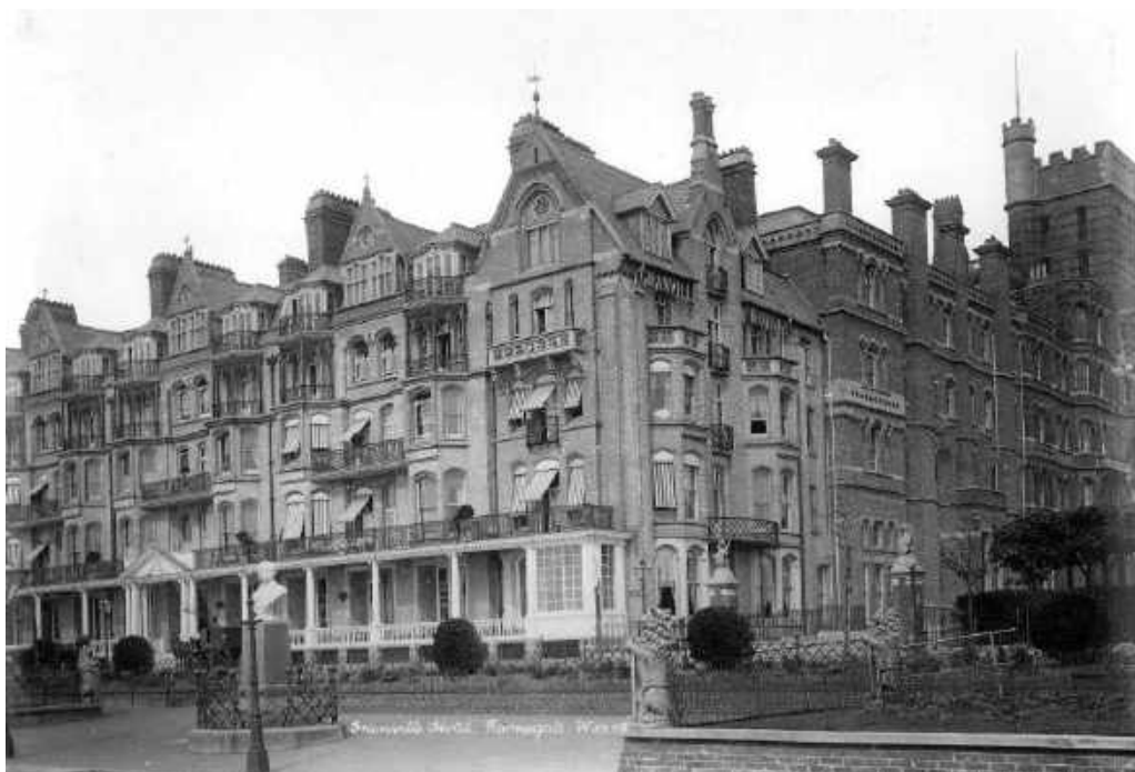
The Granville Hotel, c.1890-1910, using blinds and awnings to prevent rooms from overheating
